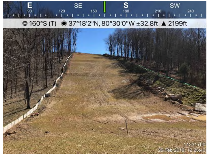
Fig. 4: STA 11501+19 – Area stabilized. Controls in place.
