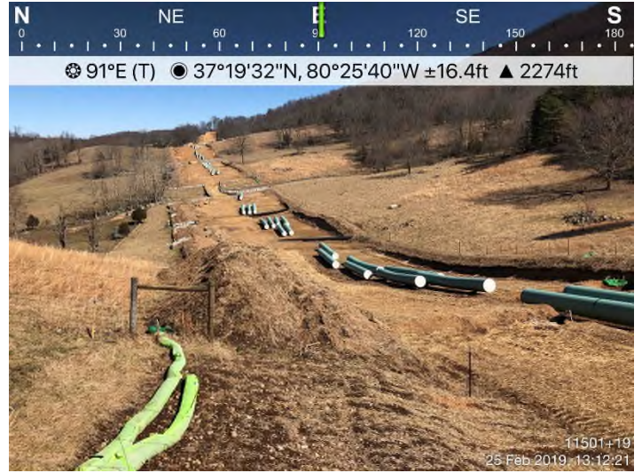
Fig. 4: STA 11501+19 – Area stabilized. Controls in place.
