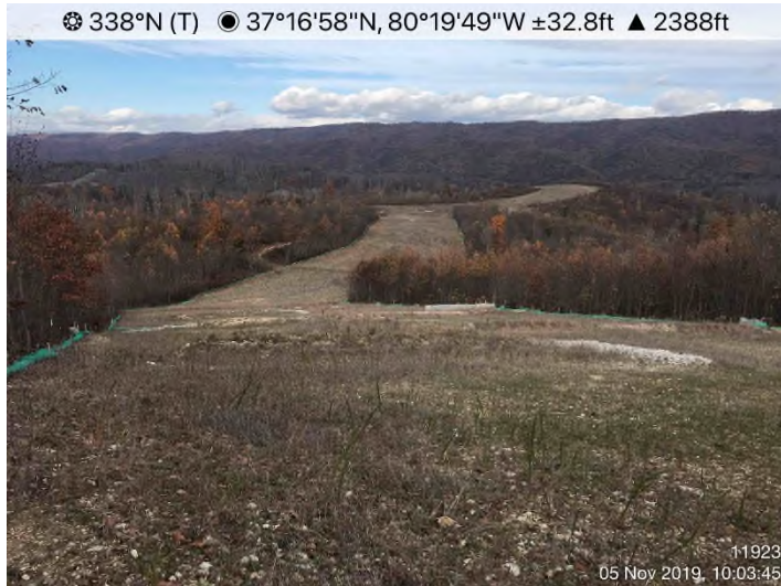
Fig. 3: STA 11865+00 – Controls in place and functioning properly. Area adequately stabilized.
