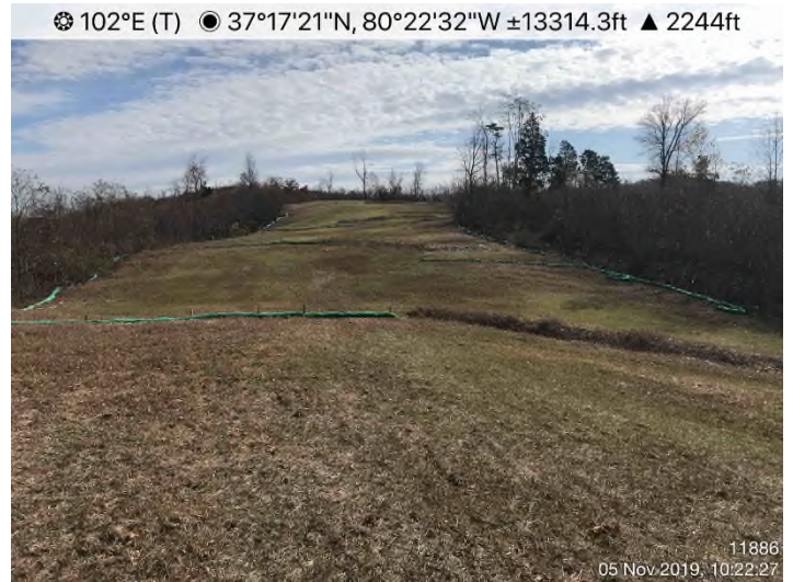
Fig. 4: STA 11795+00 – Controls in place and functioning properly. Area adequately stabilized.
