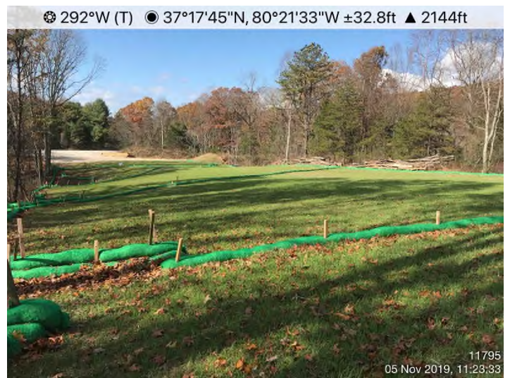
Fig. 4: STA 11795+00 – Controls in place and functioning properly. Area adequately stabilized.
