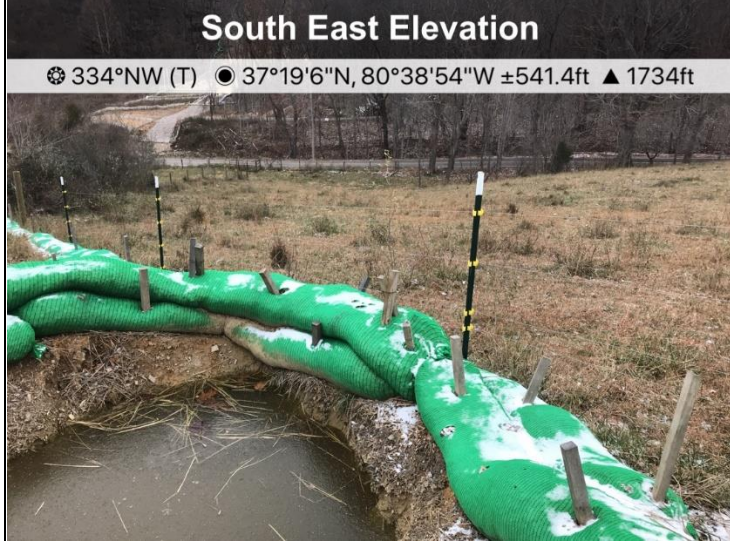
Fig. 1 At St#10933+32 no sediment observed off the ROW
