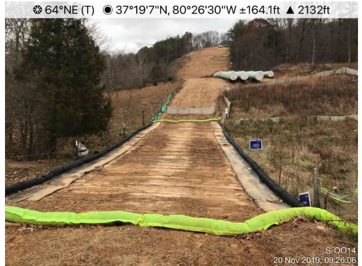
Fig. 4: STA 11327+85 – Controls in place and functioning properly along Stream S-NN12. Area adequately stabilized with straw.
