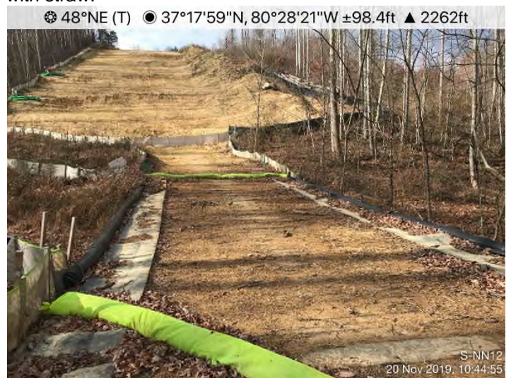
Fig. 4: STA 11327+85 – Controls in place and functioning properly along Stream S-NN12. Area adequately stabilized with straw.
