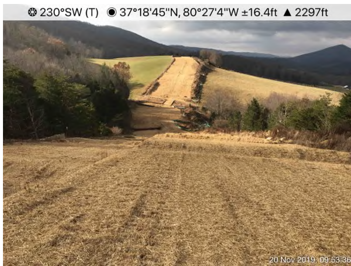
Fig. 3: STA 11412+71 – Controls in place and functioning properly. Area adequately stabilized.
