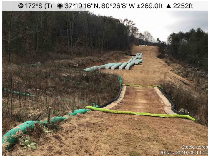
Fig. 3: STA 11412+71 – Controls in place and functioning properly. Area adequately stabilized.
