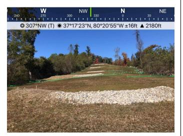
Fig. 4 Near MP 223.2 are has been stabilized.
