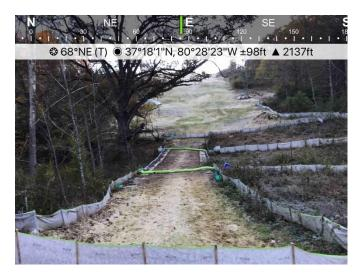
Fig. 2 Designated stream S-NN11, ECD's in place and functioning.
