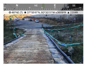
Fig. 3 Near MP 224.4 temp/ permanent waterbars have been installed
