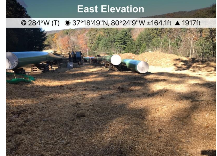
Fig. 4 St#11600-11613 has been adequately mulched.
