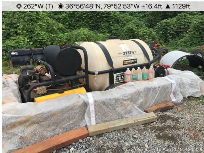
Fig. 3: Laydown Yard 032 – Secondary containment structure in place and functioning.
