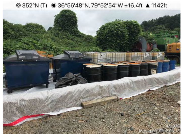
Fig. 4: Laydown Yard 032– Secondary containment structure in place and functioning.
