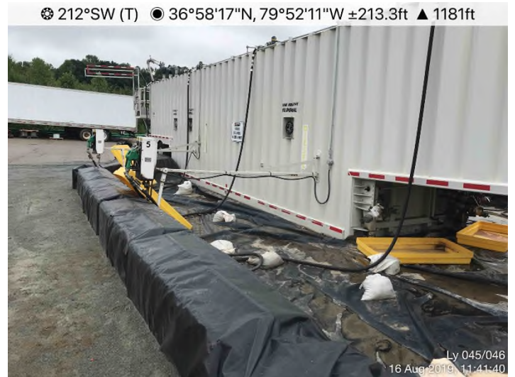
Fig. 4: Laydown Yard 032– Secondary containment structure in place and functioning.
