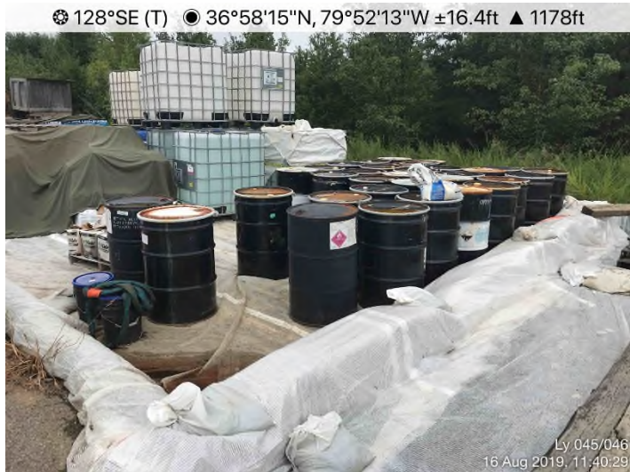
Fig. 3: Laydown Yard 032 – Secondary containment structure in place and functioning.
