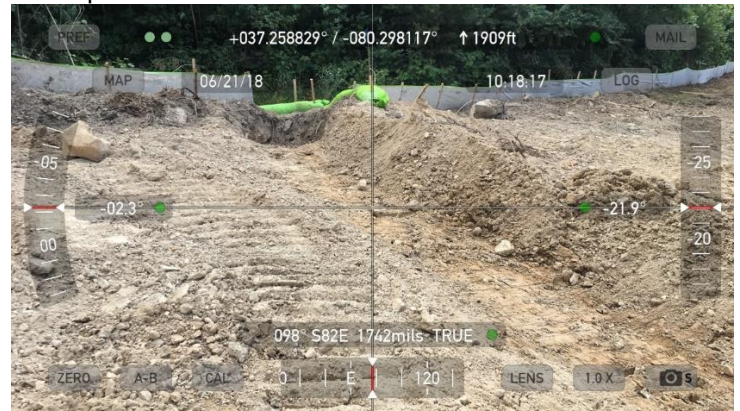
Fig. 2 Description: Water bar
