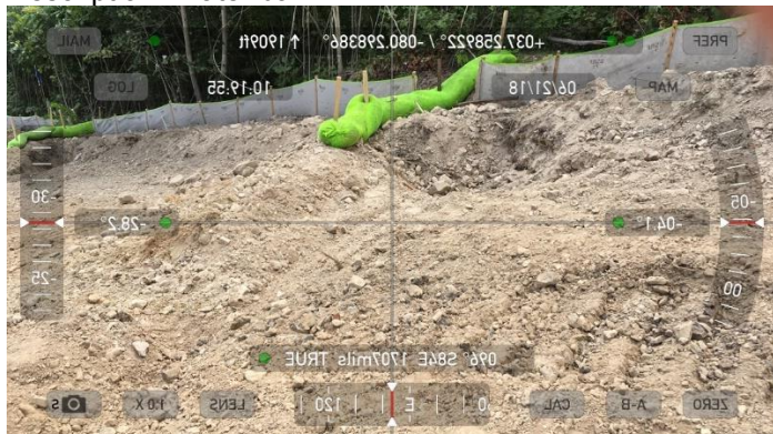
Fig. 3 Description: Water bar
