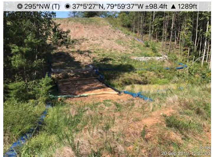
Fig. 4: Stream S-II8 – Controls in place and area stabilized.
