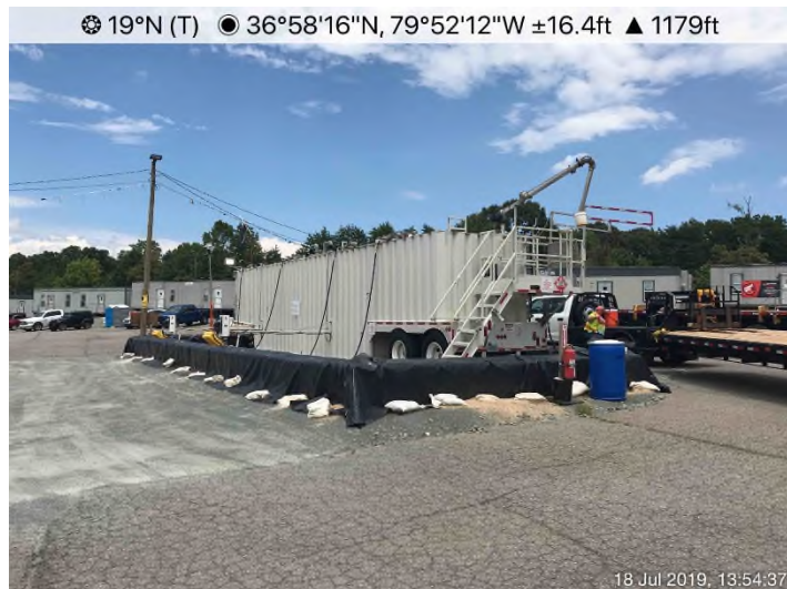
Fig. 3: Laydown Yard 045/046 – Fueling station controls in place and properly functioning.
