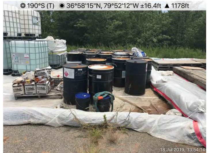
Fig. 4: Laydown Yard 045/046 – Secondary containment structure in place and functioning properly.
