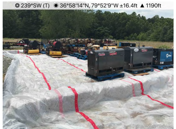
Fig. 4: Laydown Yard 045/046 – Secondary containment structure in place and functioning properly.
