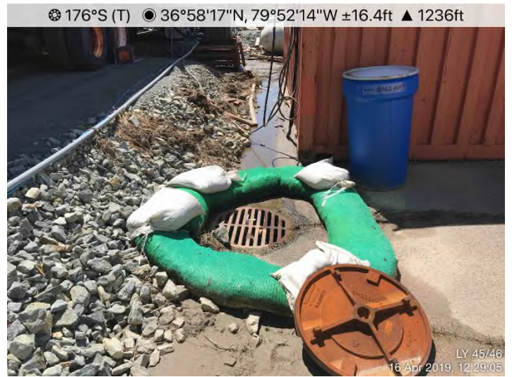
Fig. 4: LY 045/046 – Inlet protection in place.
