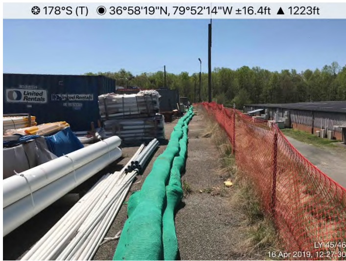
Fig. 3: LY 045/046 – Perimeter controls in place.
