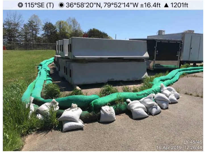
Fig. 4: LY 045/046 – Inlet protection in place.
