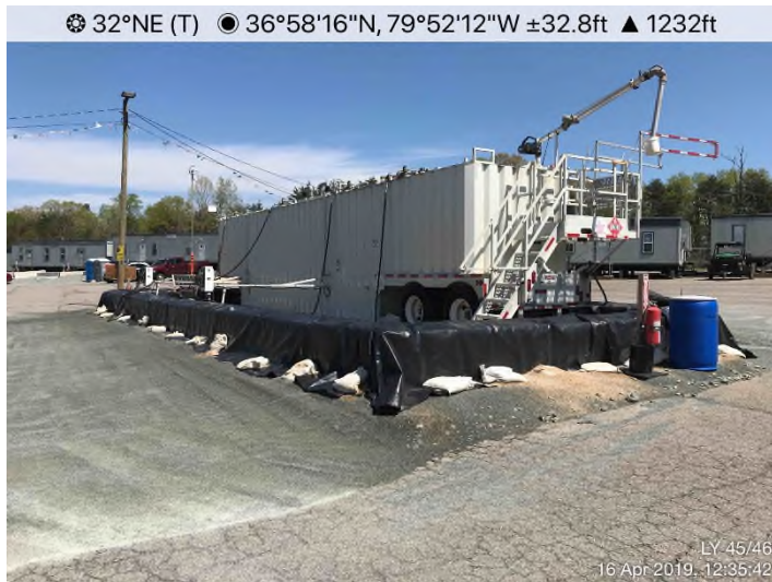
Fig. 3: LY 045/046 – Perimeter controls in place.
