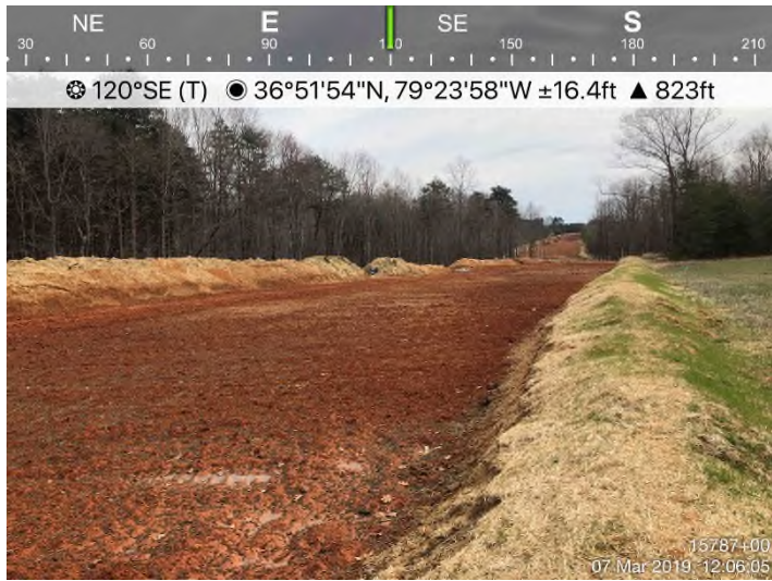
Fig. 3: STA 15787+00 – Area stabilized with Earth Guard. Controls in place.
