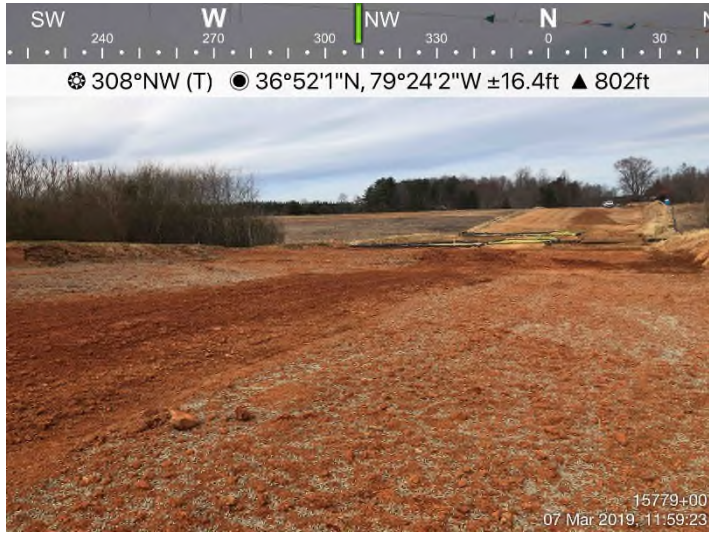
Fig. 3: STA 15787+00 – Area stabilized with Earth Guard. Controls in place.
