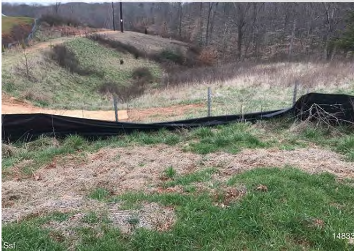
Figure 3: STA 14833+00 – SSF maintenance needed.
