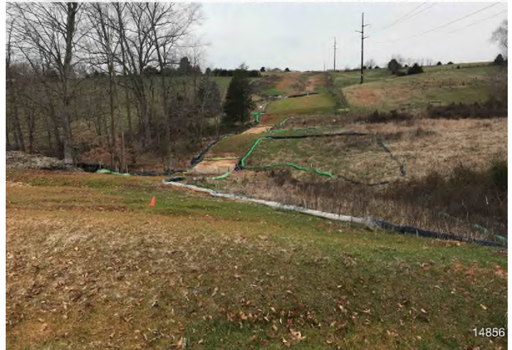
Figure 4: STA 14856+00 – Controls in place and functioning properly.
