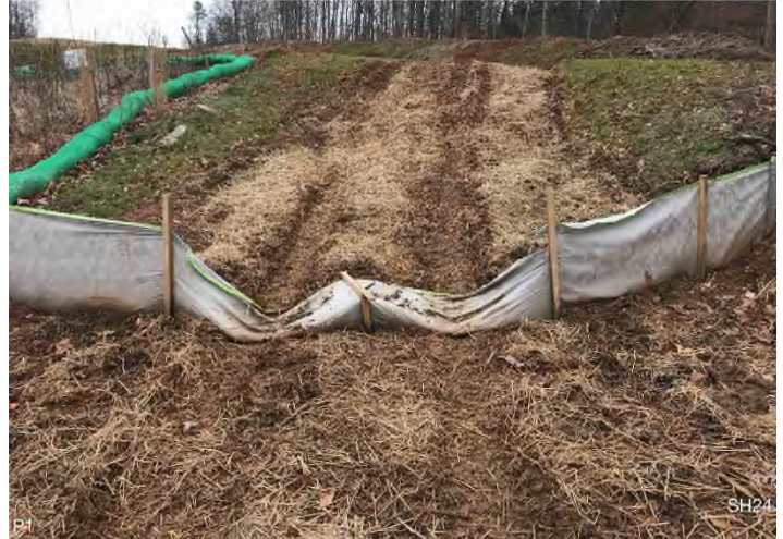
Figure 4: STA 14856+00 – Controls in place and functioning properly.
