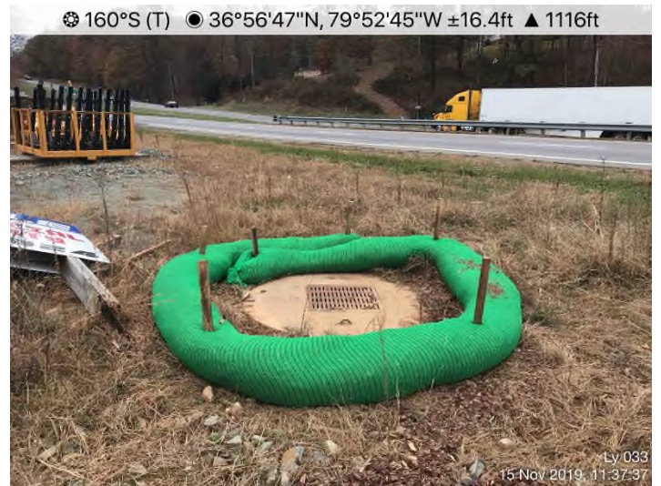
Fig. 4: Laydown Yard 033 – Controls in place around drop inlet and functioning properly.
