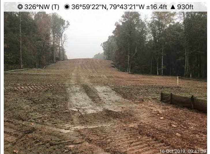
Fig. 4: STA 14656+37 – Controls in place and area stabilized with hydraulic mulch.
