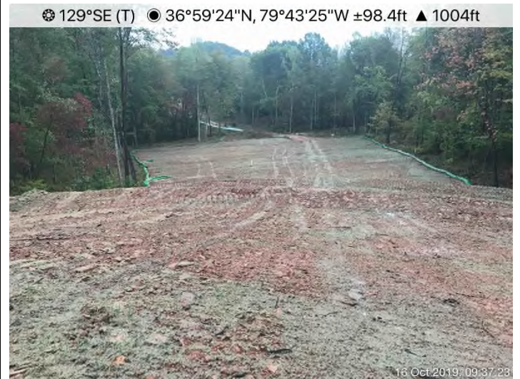
Fig. 4: STA 14656+37 – Controls in place and area stabilized with hydraulic mulch.
