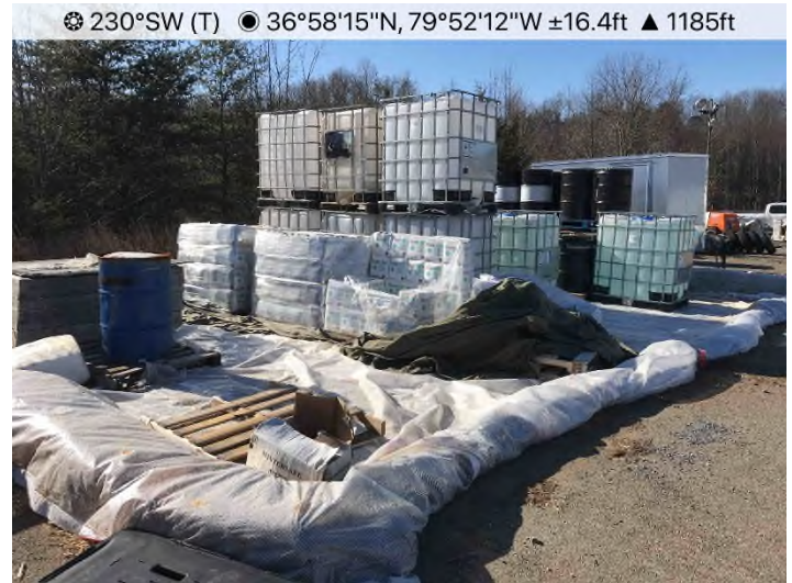
Fig. 4: Laydown Yard 032 – Secondary containment in place and functioning properly.
