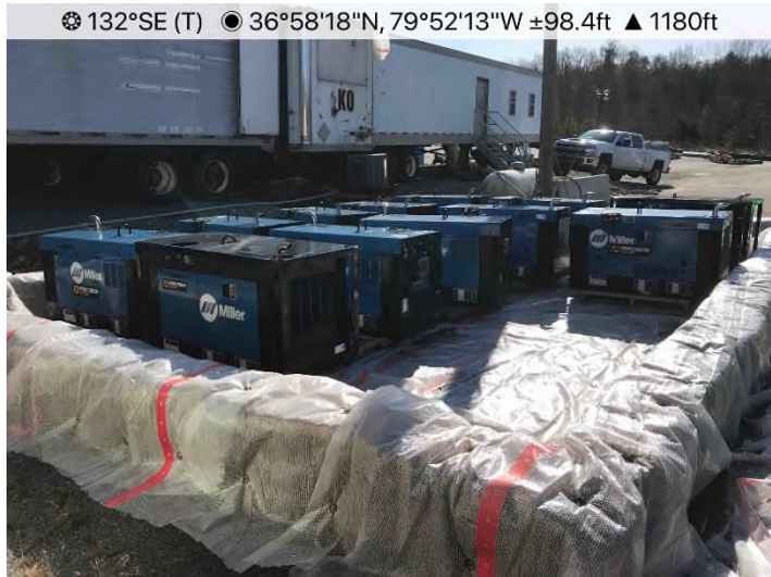
Fig. 3: Laydown Yard 045/046 – Secondary containment in place around fueling station and functioning properly.
