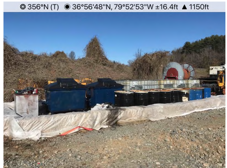
Fig. 4: Laydown Yard 032 – Secondary containment in place and functioning properly.
