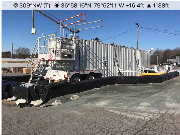
Fig. 3: Laydown Yard 045/046 – Secondary containment in place around fueling station and functioning properly.
