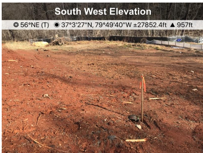
Fig. 3 Between St#14235+00 and St#1428 is not adequately stabilized.
