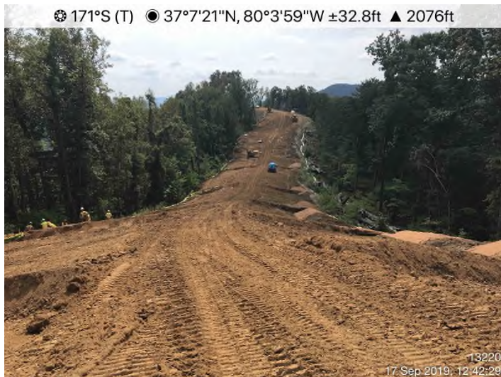
Fig. 3: STA 13220+00 – Winter stabilization grading in progress.
