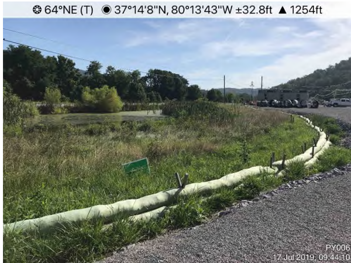
Fig. 3: Pipe Yard 006 – Secondary containment in place and functioning properly.
