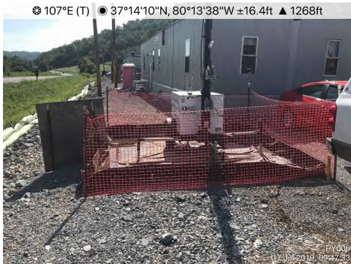
Fig. 3: Pipe Yard 006 – Secondary containment in place and functioning properly.
