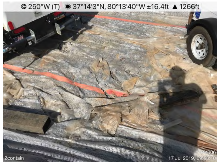
Fig. 4: Pipe Yard 006 – Secondary containment requires maintenance.
