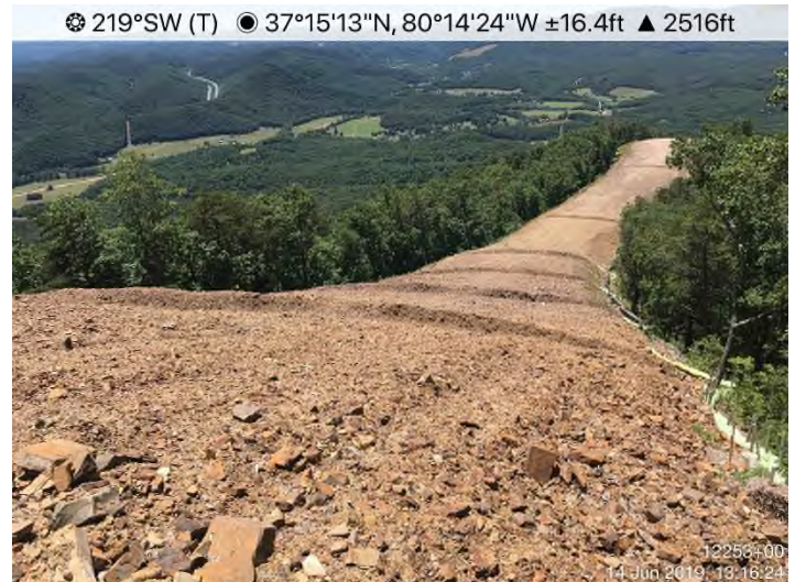
Fig. 4: STA 12252+00 – Controls in place. Area stabilized with Earth-Guard.
