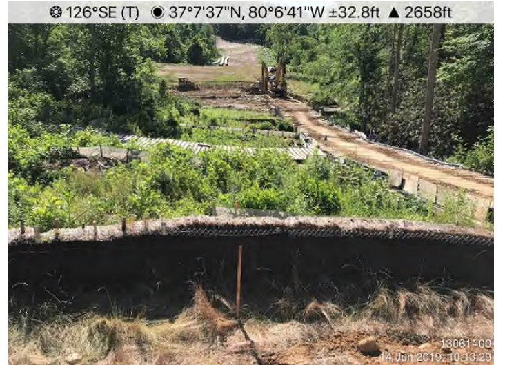
Fig. 4: STA 12252+00 – Controls in place. Area stabilized with Earth-Guard.
