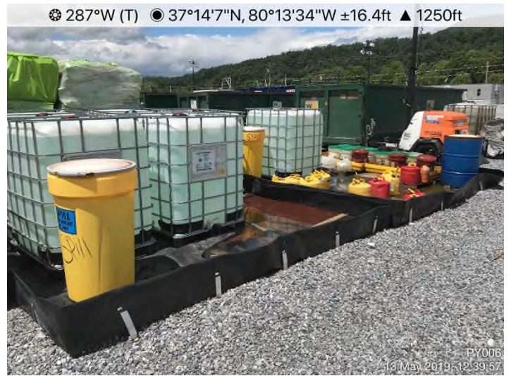
Fig. 4: PY-006 – Secondary containment controls in place.
