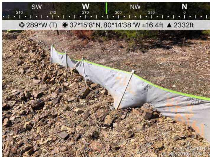
Fig. 8: STA 12240+81 – P1 needs maintenance.
