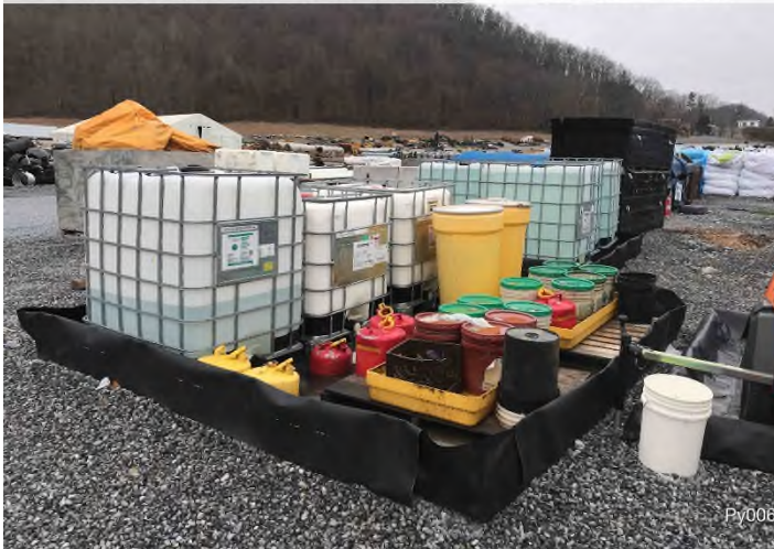
Figure 3: Pipe Yard 006 – Secondary containment in place and functioning properly.
