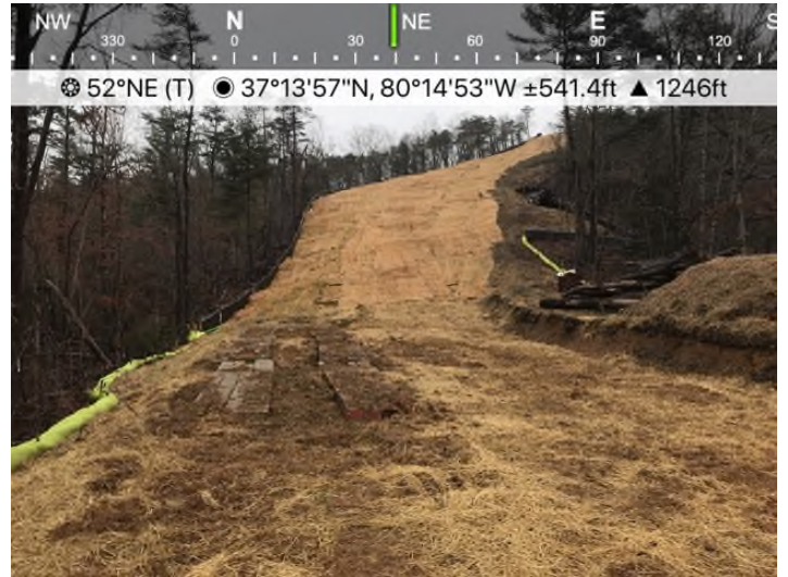
Fig. 4: STA 12098+44 – Temporary crossing for S-MM13 adequately maintained.
