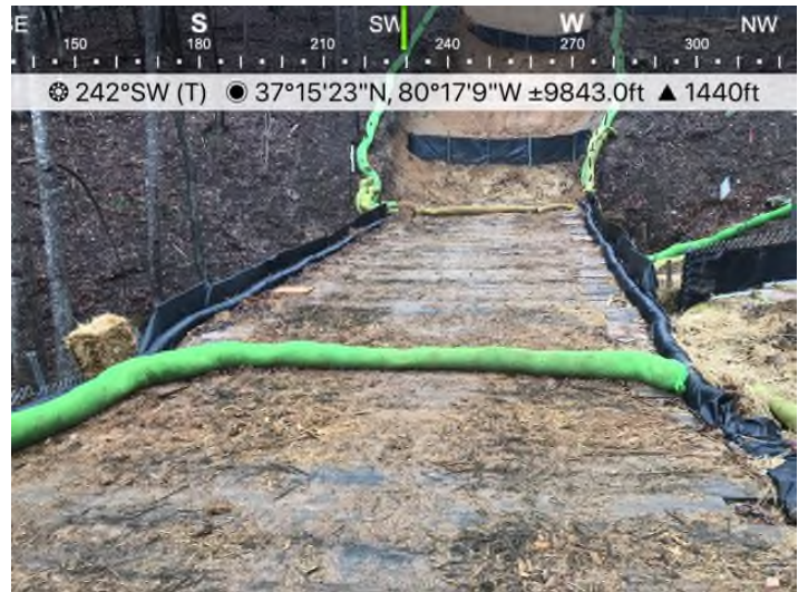
Fig. 4: STA 12098+44 – Temporary crossing for S-MM13 adequately maintained.
