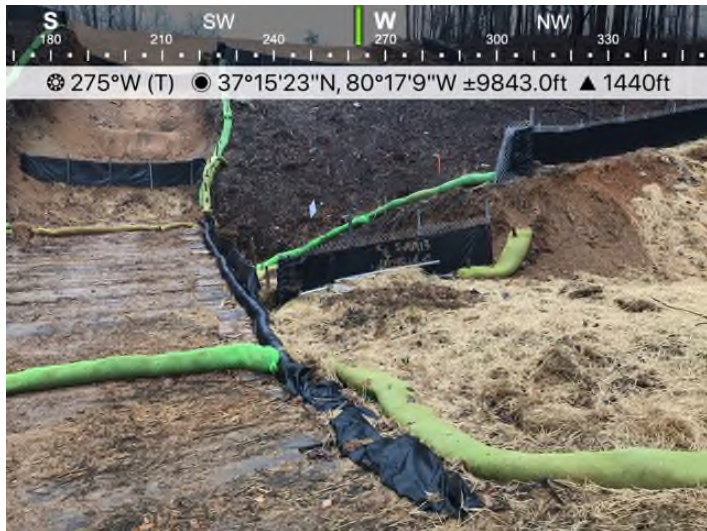
Fig. 3: STA 12098+44 – ECDs installed and maintained around S-MM13.
