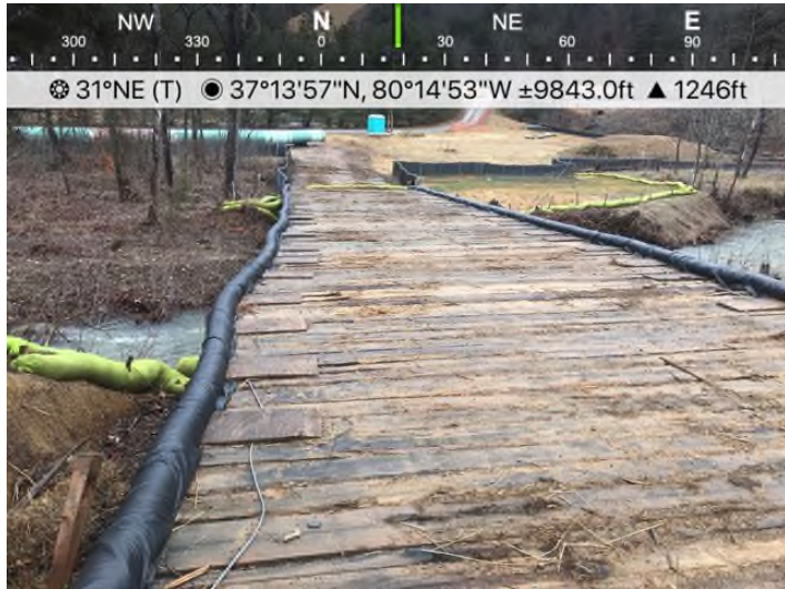
Fig. 3: STA 12098+44 – ECDs installed and maintained around S-MM13.
