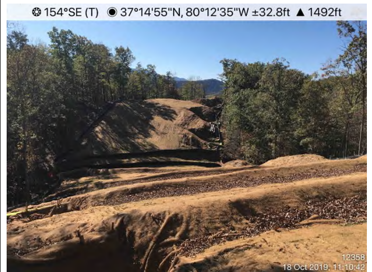
Fig. 4: STA 12358+00 – Controls in place and area stabilized with matting and straw.
