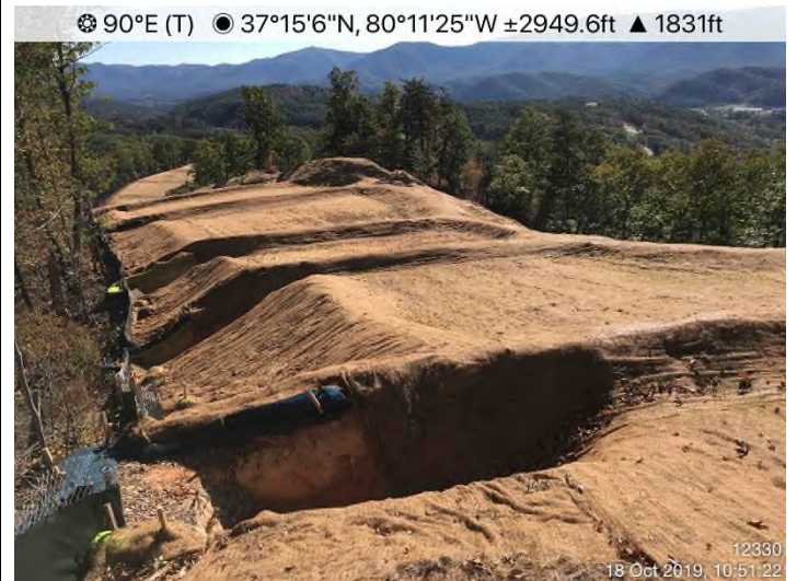
Fig. 4: STA 12358+00 – Controls in place and area stabilized with matting and straw.
