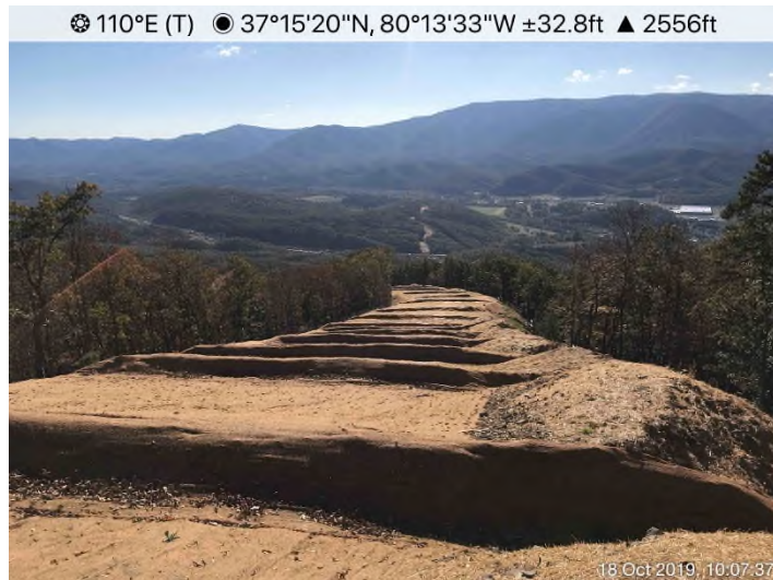
Fig. 3: STA 12341+00 – Controls in place and area stabilized with matting and straw.
