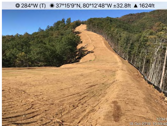
Fig. 3: STA 12341+00 – Controls in place and area stabilized with matting and straw.
