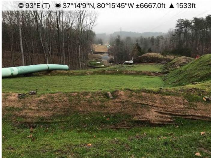
**Fig. 2: STA 12116+00** – Controls in place and functioning properly. Area stabilized.
