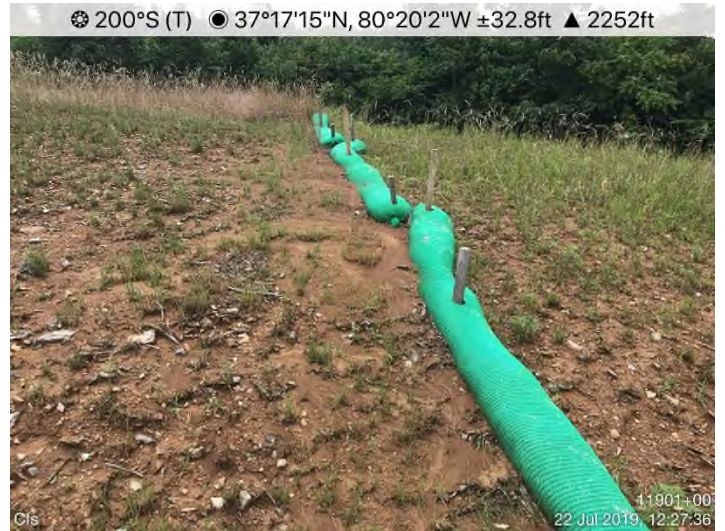
Fig. 4: STA 11903+00 – CFS maintenance needed.
