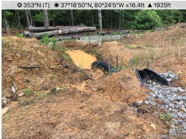
Fig. 3: STA 11901+00 – CFS maintenance needed.
