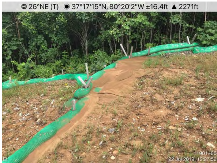
Fig. 3: STA 11901+00 – CFS maintenance needed.
