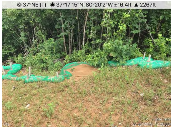
Fig. 6: STA 11901+00 – CFS maintenance needed.
