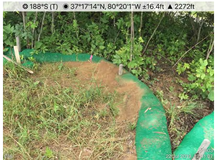
Fig. 4: STA 11903+00 – CFS maintenance needed.
