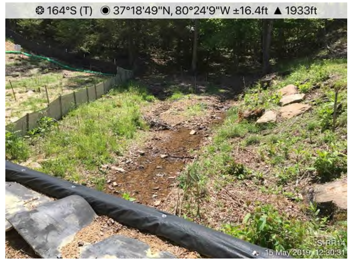
Fig. 8: Stream S-RR14 – Controls in place.
