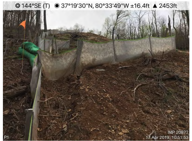
Fig. 4: STA 10991+00 – P1 undermined.
