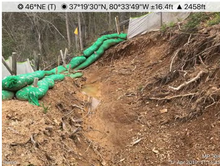
Fig. 7: STA 11025+00 – Area adequately stabilized. Controls in place.
