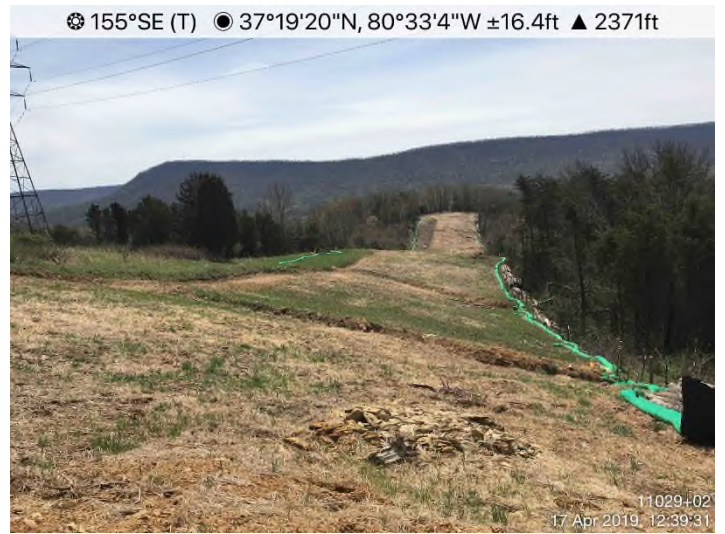
Fig. 8: STA 11029+02 – Area adequately stabilized. Controls in place.
