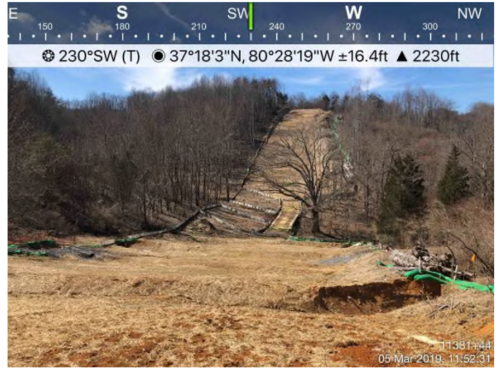
Fig. 6: STA 11381+44 – Area adequately stabilized. Control in place.
