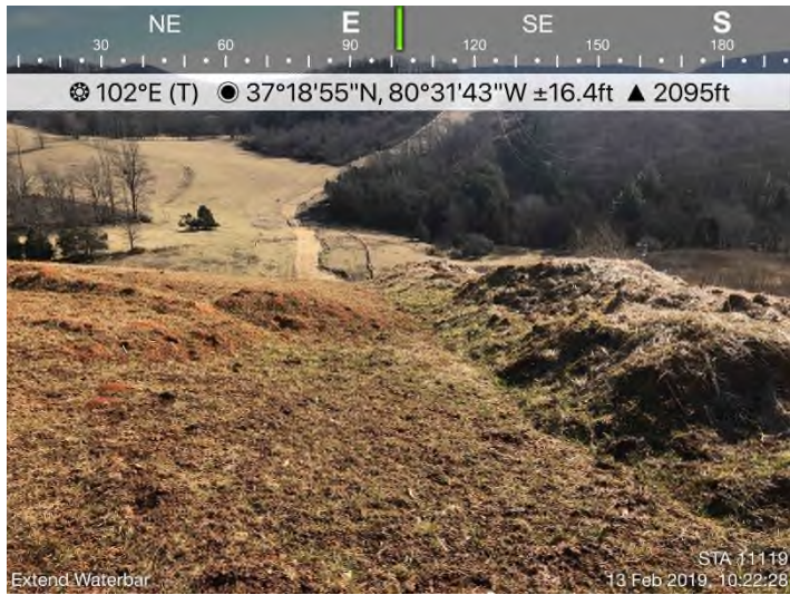
Fig. 3: STA 11119 – Waterbar does not extend to edge of LOD.
