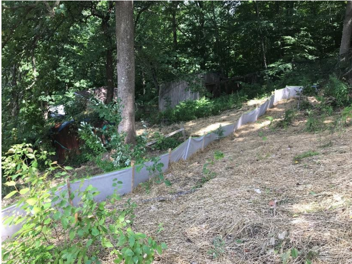
Stabilized area off of ROW with silt fence.
