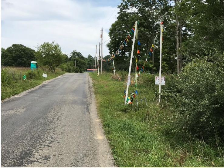
Portable toilet located well-away from stream.
