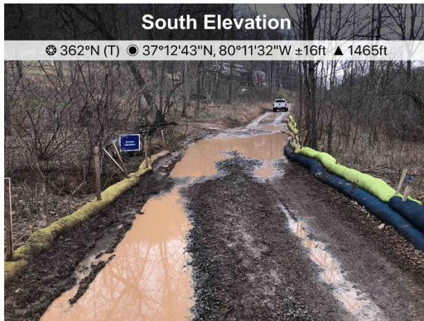
Figure 1: ECD's are installed and functioning along access road MN 278.01 and designated stream S-EF54A.
