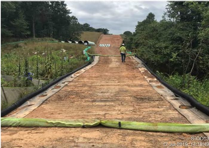
Fig. 4: **STA 11432+00** – Sump maintenance needed.
