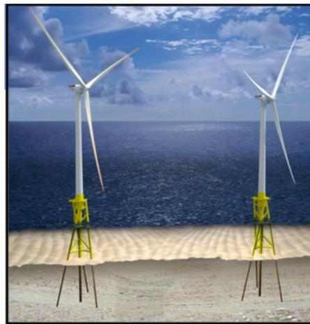
*Beneath the surface: This graphic illustrates the proposed foundations for the two VOWTAP turbines. Specific foundation types for the commercial project have not yet been identified.*
