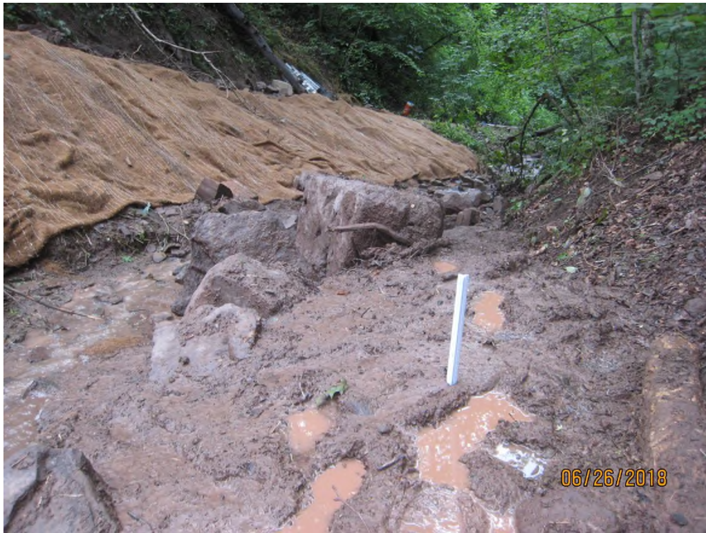
Photo 1: Sedimentation within "Stream 39" ~25' downstream of LOD Orientation: Downstream
